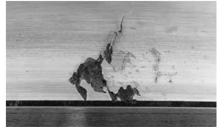
Fig. 1: Point Surface Origin (PSO) spalling
