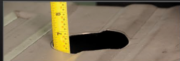
Cut foam 1in TALLER than tank depth
