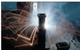
Precision robotic welding for superior strength and fit
