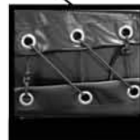
Grommets away from frame eliminates contact wear
