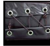
Grommets away from frame eliminates contact wear
