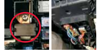
Figure 12 ELD bottom fuse box
